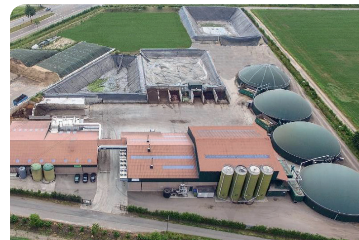
Site Biogas Bree
